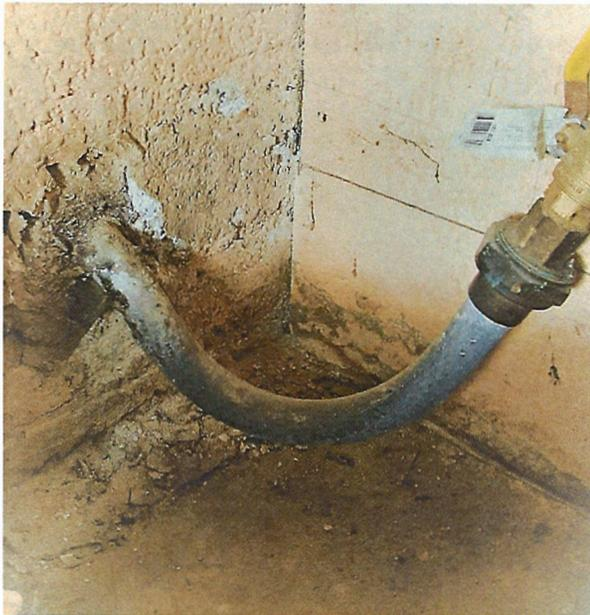
*Photo of a lead service line in a home in North Platte, NE.*
